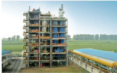
常压气流床煤制气装置点火运行 The atmospheric pressure entrained-flow gasification equipment launched.
